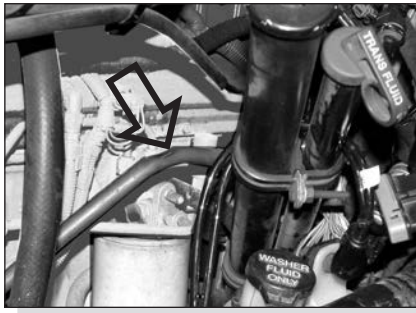
Damaged discharge line shown.
